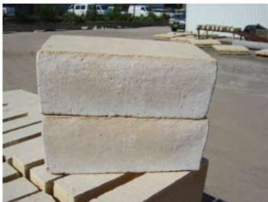
Blocks with Efflorescence
