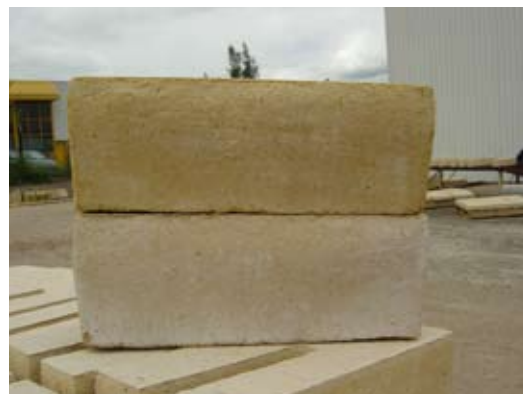
Cleaned with Enviro Pacific Efflorescence Remover
